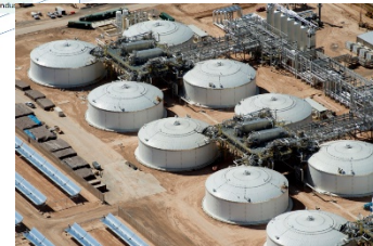
Solana CSP plant (US)
